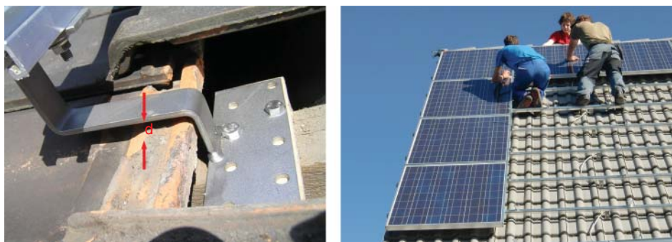
Figure 6.34 Fixing the on-roof system: The roof hooks are screwed to the rafters and thus form the base for holding the module supports. A sufficient distance between roof hooks and roof tiles is important in order to avoid damaging the tiles. Source: Ch. Niemann, A. Schroer.
