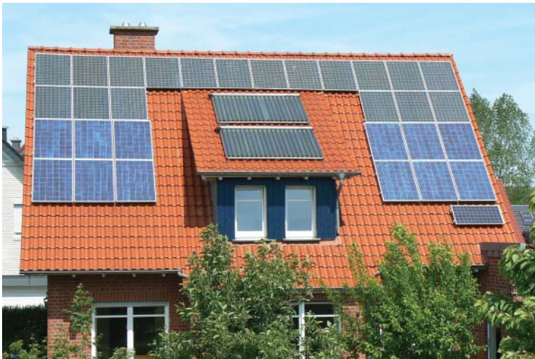
Figure 6.33 On-roof system on a private house: There should be at least one row of tiles spacing at the side in order to reduce the possibility of attack by the wind.
