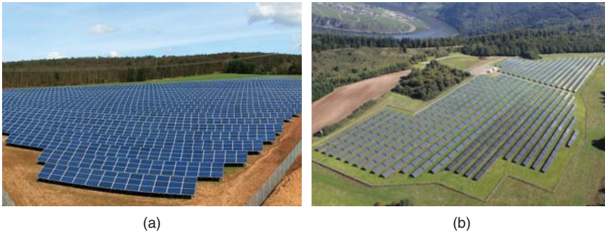
Figure 6.26 View of two solar power plants: (a) Citizen's solar power plant at Hofbieber-Traisbach with 1.3 MWp of multicrystalline modules. Source: IBC SOLAR AG. (b) 3.5 MWp solar power plant at Mehring on the Moselle with CdTe modules. Source: juwi Solar GmbH.
